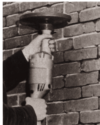
Illustration 15 – Tuck pointing using a reinforced organic bonded abrasive wheel
